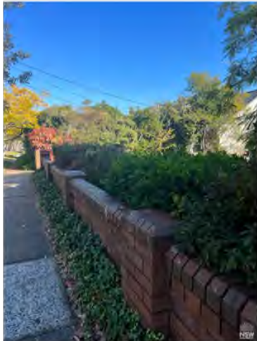
Caption: Roseville Avenue street fencing (northern side)
