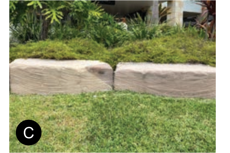
C Sandstone retaining wall
