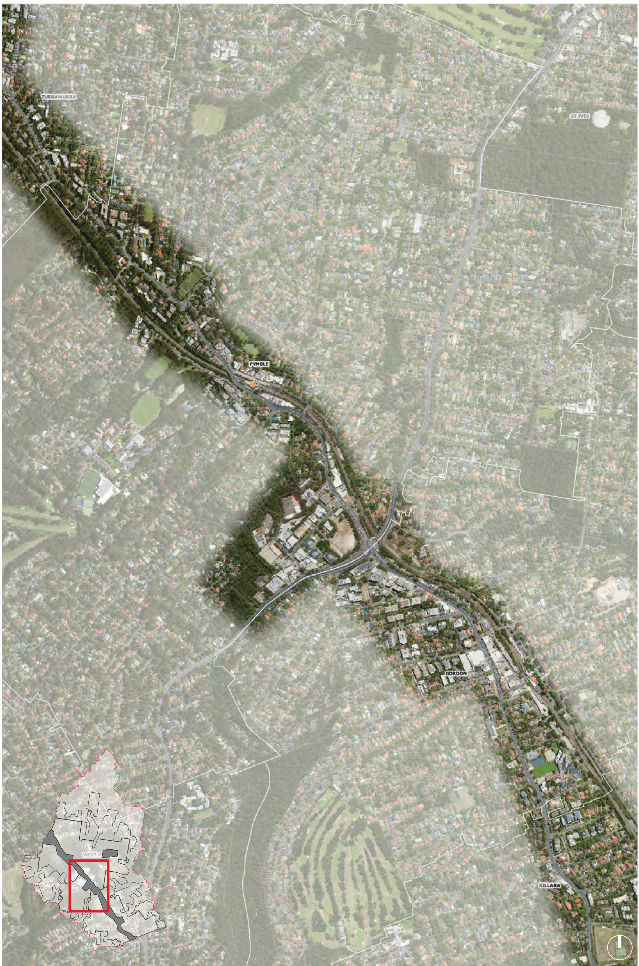
Figure 19: Pymble and Gordon Centres along Pacific Highway
