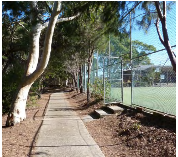
Plate 1.34: Typical concrete path
