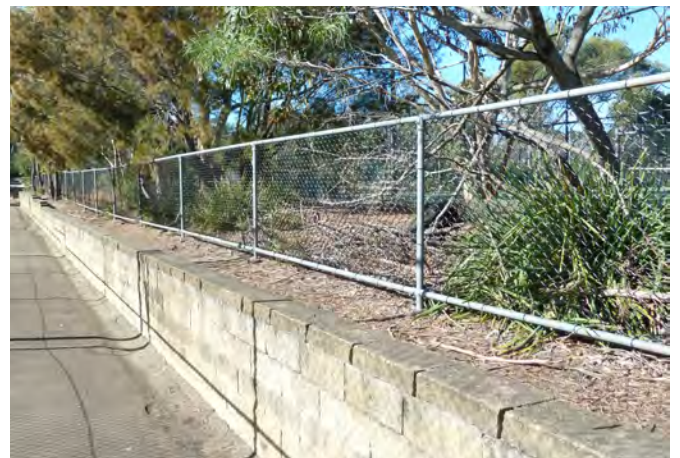
Plate 1.13: Typical retaining walls with fencing on the site
