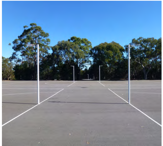
Plate 1.5: Primary netball courts on asphalt
