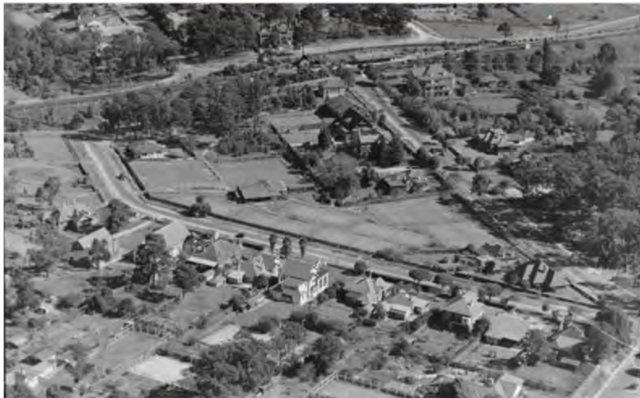
Above Killara, Arnold Street, and station in approximately 1933-34. (Source: State Library, https://collection.sl.nsw.gov.au/record/nGm303Y )
