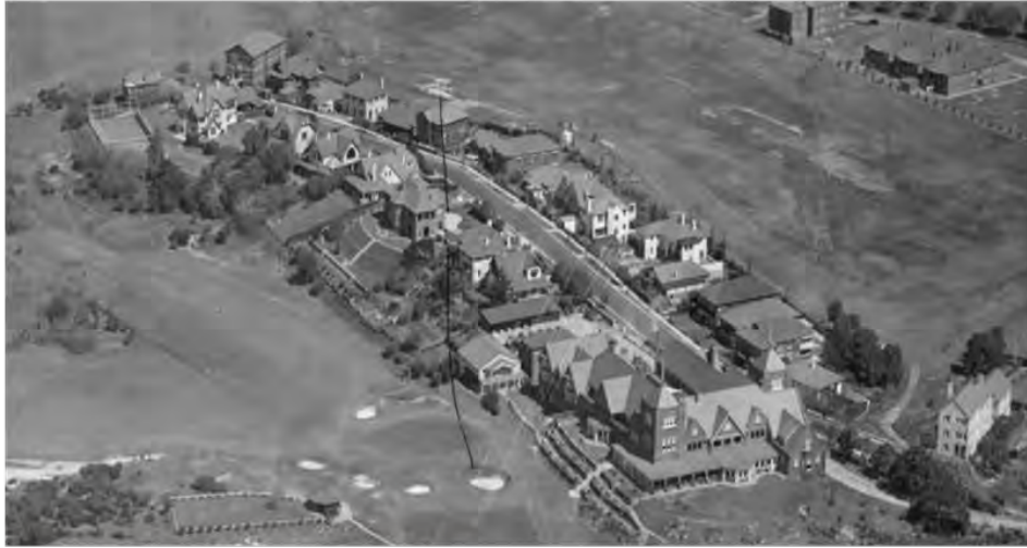
Above: Kent Road – Rose Bay – in 1940s (Source: State Library, https://collection.sl.nsw.gov.au/record/114dZbe1 )
