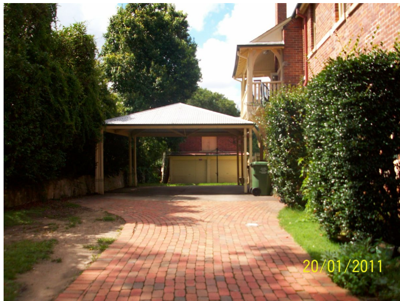
Figure 2: The existing carport on the western side of the house
