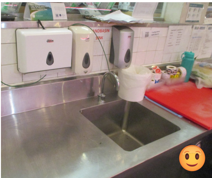
Supply hand basins with pump soap, warm water and single use paper towels
